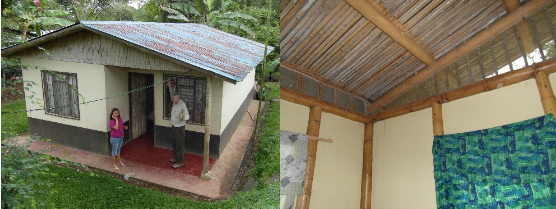
Figure 6. National bamboo project housing in Milano, Costa Rica – photos taken at 20+ years since construction (Kaminski, 2012).
